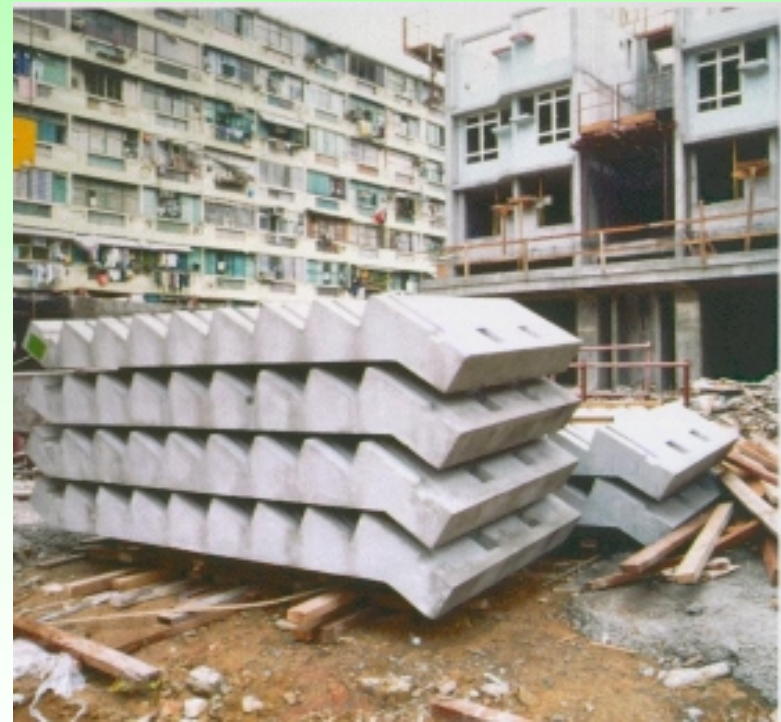
預製樓梯 Prefabricated stair flights
