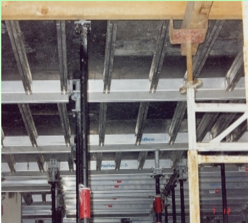
系統板模 System formwork
