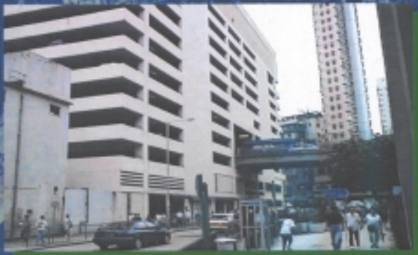
油麻地多層停車場大樓 Yau Ma Tei Multi-Storey Car Park Building
