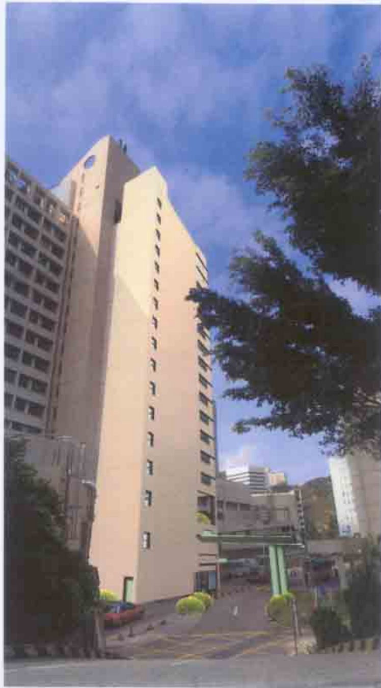
從東面望向工程完成後的新升降機樓外觀(模擬圖) VIEW OF BLOCK S FROM EAST DIRECTION UPON COMPLETION (ARTIST'S IMPRESSION)
