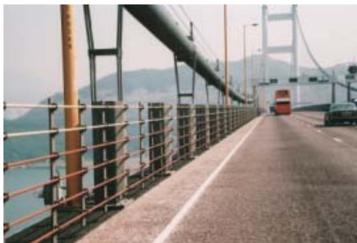
Figure 9.6 – Tensioned Steel-strand P4 parapet of the Tsing Ma Bridge
