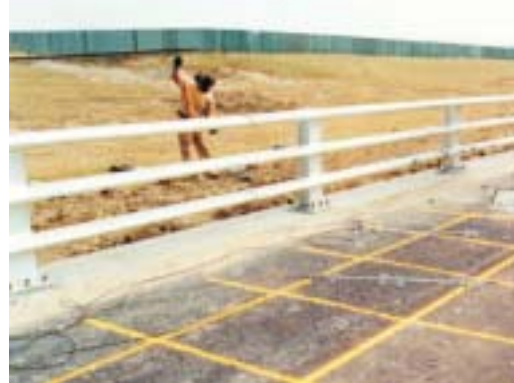
Figure 9.9 – Modified P1 aluminium parapet
