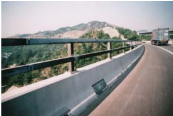
Figure 9.7 – Ting Kau viaduct
