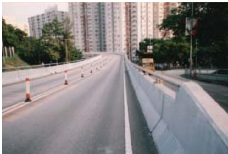
Figure 9.4 – Concrete P1 parapet with a metal railing
