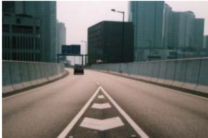
Figure 9.5 – High containment P4 concrete parapet
