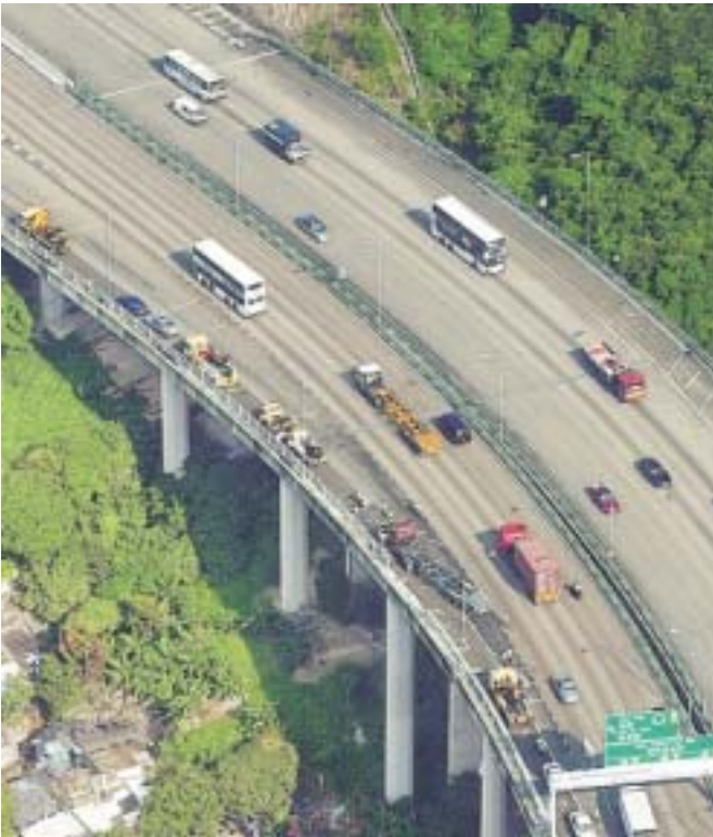
Figure 3.5 – An aerial photo of Tuen Mun Road at the location of incident (by courtesy of Ming Pao)
