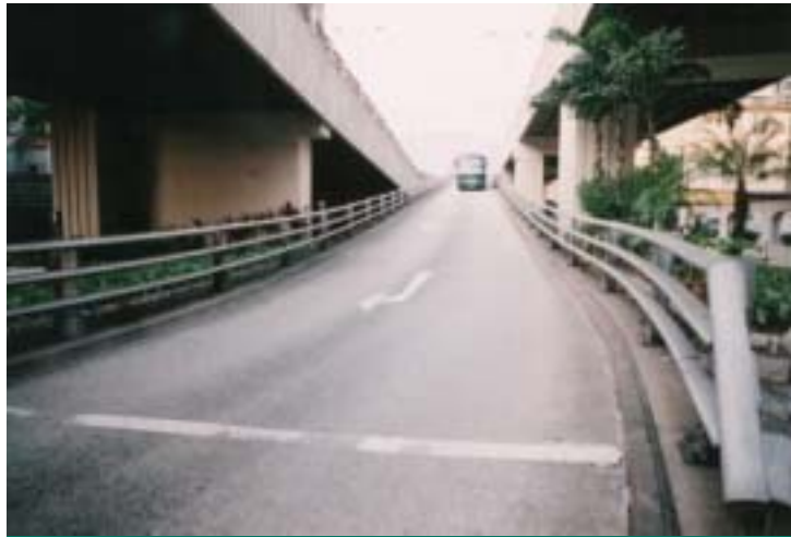
Figure 9.3 – First generation P1 3-rail aluminium parapet
