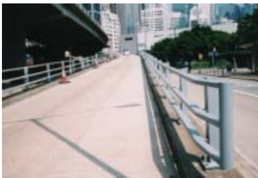
Figure 9.8 – Modified P1 steel parapet
