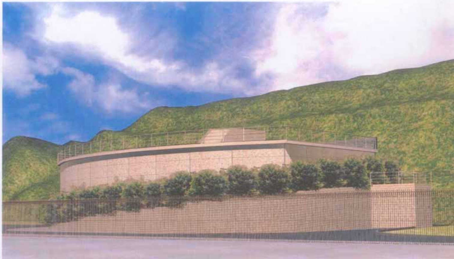
擬建的九肚高地食水配水庫 THE PROPOSED KAU TO HIGH LEVEL FRESH WATER SERVICE RESERVOIR
