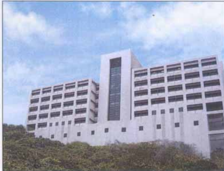
專科門診大樓南面立面圖 (改善工程前) South Elevation of the Specialist Outpatient Block (Before Improvement)
