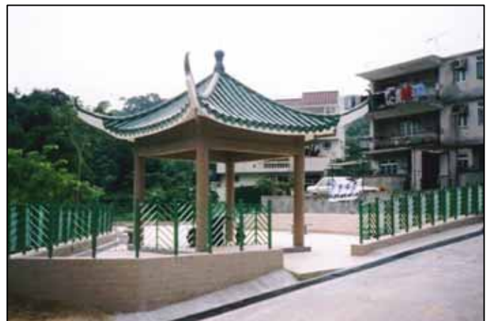
改善工程後 After Improvement works
