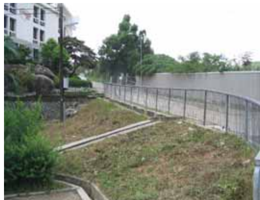
清理後 After operation
