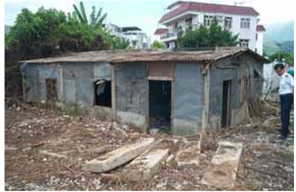
清理後 After operation
