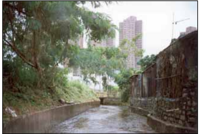
清渠及剪草後 After desilting & grass cutting
