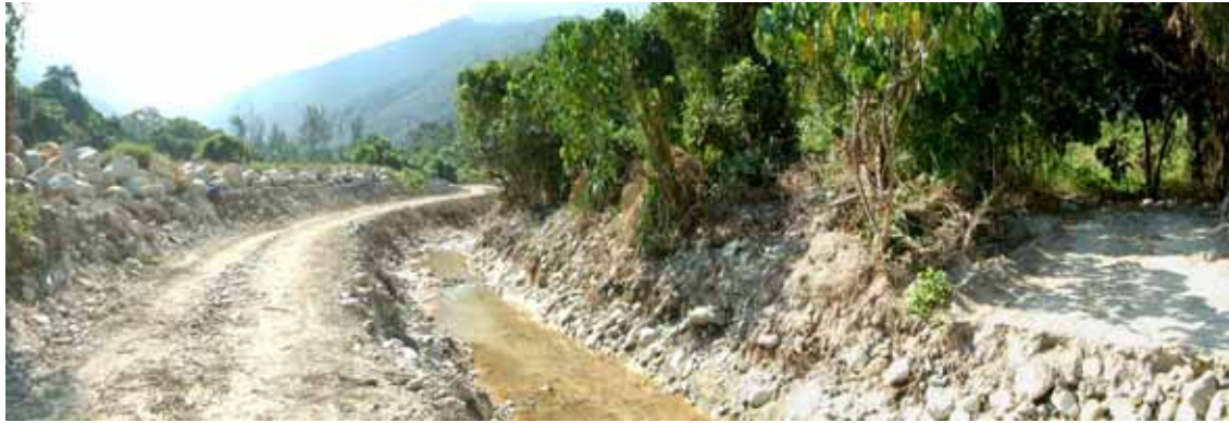
(a) After excavation (before reinstatement) (7 November 2003)
