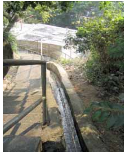
清理後 After operation
