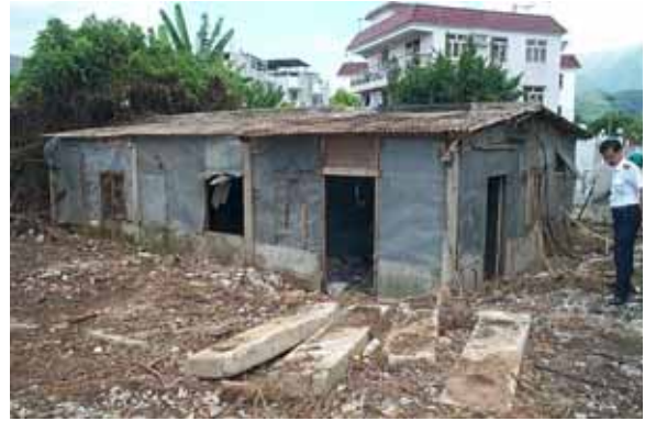
清理後 After operation
