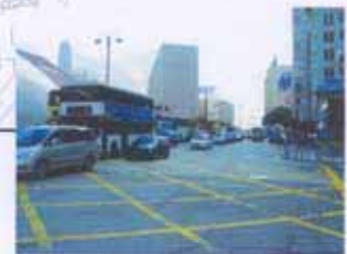
Pedestrian Crossings Requiring Improvement
