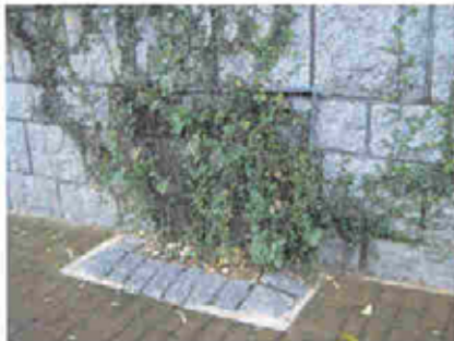
牆腳花槽種植攀緣植物 Climber Planting in Toe Planter
