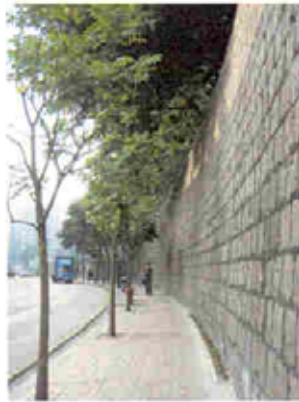
樹槽植樹 Tree Planting in Tree Pit
