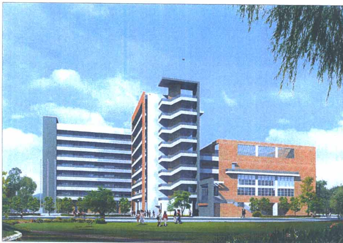
從北面望向第1所小學校舍的構思圖 VIEW OF THE PREMISES OF FIRST PRIMARY SCHOOL (325EP) FROM NORTHERN DIRECTION (ARTIST'S IMPRESSION)
