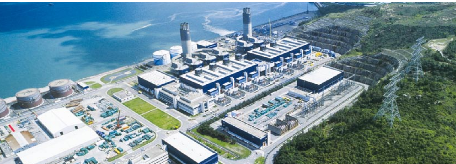
Black Point Power Station: built by private sector investment to provide clean power to our community for a quarter of a century and beyond
