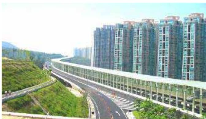
Partial noise enclosures along section of Ma On Shan Bypass near Monte Vista.
