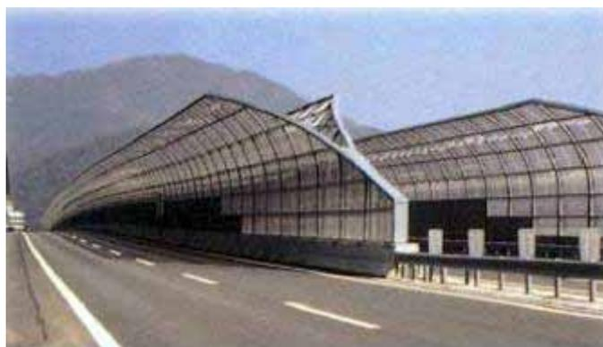
An example of light weight noise barriers using aluminum frame and polycarbonate plate.
