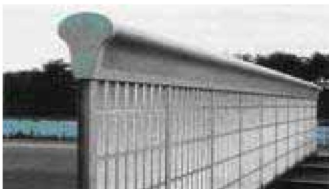
Sound absorbing device attached on the top edge of a noise barrier.
