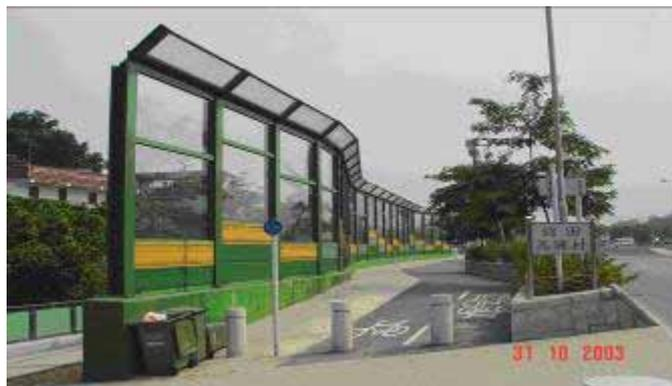
An example of noise barriers constructed with relatively light materials and a design blending with the surrounding environment, locating at Kam Tin Road near the junction to Tsing Long Highway.
