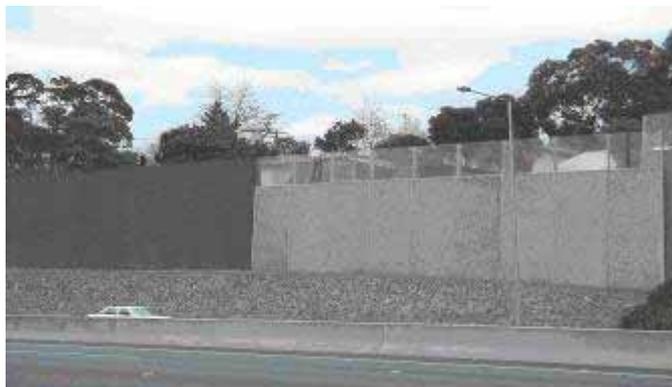
Tall concrete and acrylic barriers used to protect residences from heavily-trafficked freeway and also reduce over-shadowing of residences.
