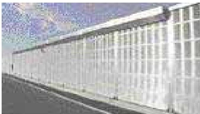
Active soft edge noise barriers installed in Japan.
