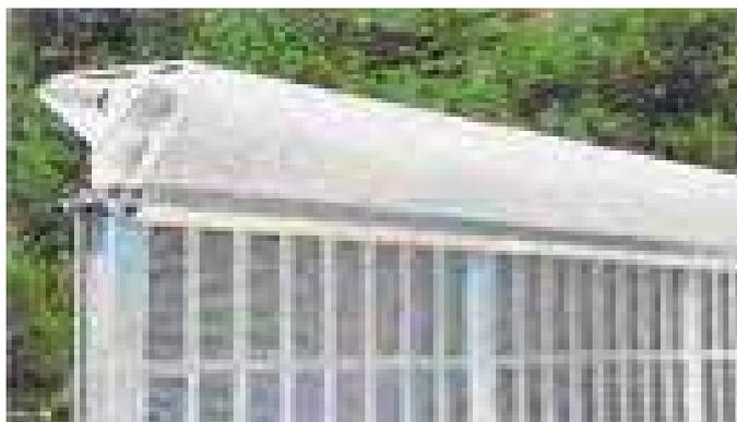
Multi-diffraction sound-absorbing noise barriers produced in Japan.
