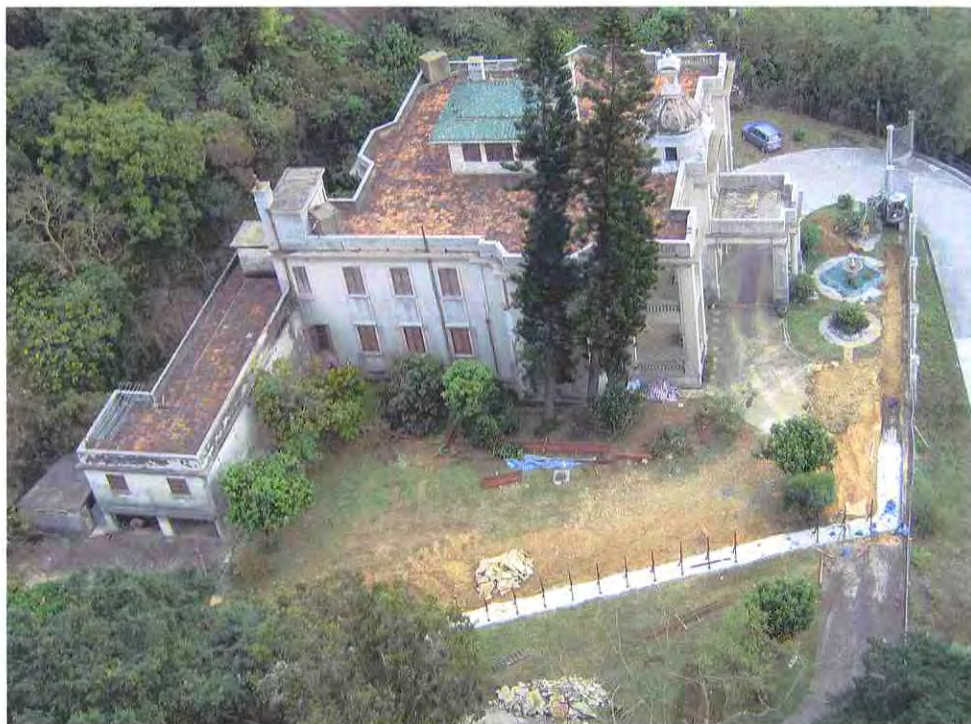
Bird's eye view of the Building, its annex block, the fountain (right) and the greenery in the immediate environ.
