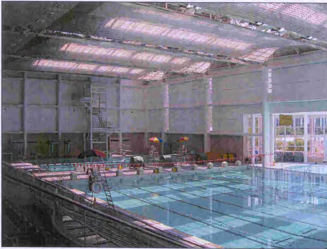
Improvement to Kowloon Park Swimming Pool (Before) 九龍公園游泳池改善工程 (工程前)
