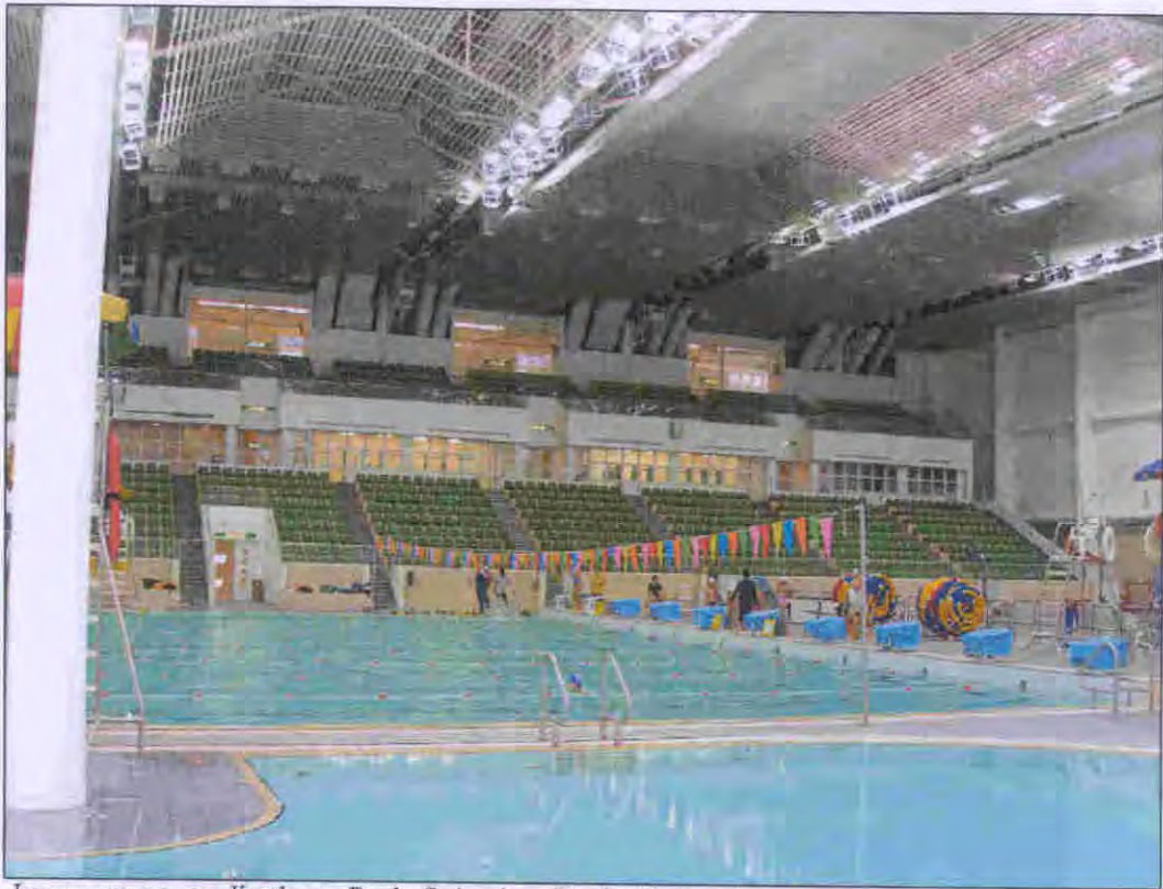
Improvement to Kowloon Park Swimming Pool (Before) 九龍公園游泳池改善工程 (工程前)
