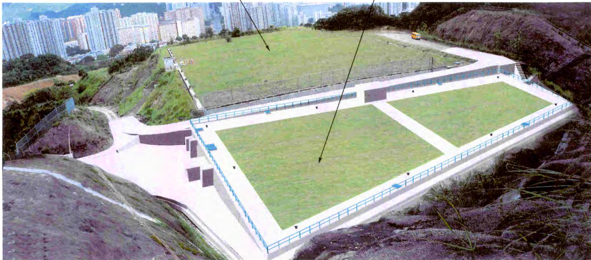
擬建的多石海水配水庫 PROPOSED TO SHEK SALT WATER SERVICE RESERVOIR
