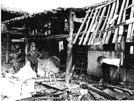
Collapse of old wood structure house
