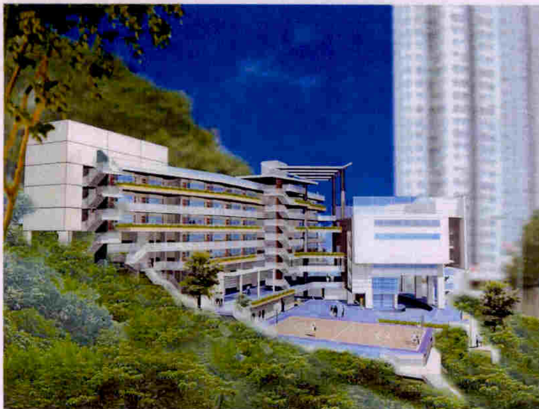
VIEW OF THE SCHOOL PREMISES FROM SOUTH-WESTERN DIRECTION (ARTIST'S IMPRESSION) 從西南面望向校舍的構思圖
