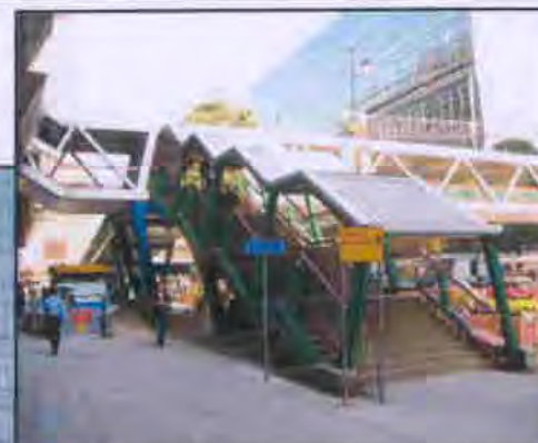
現有行人天橋樓梯 EXISTING FOOTBRIDGE STAIRCASE
