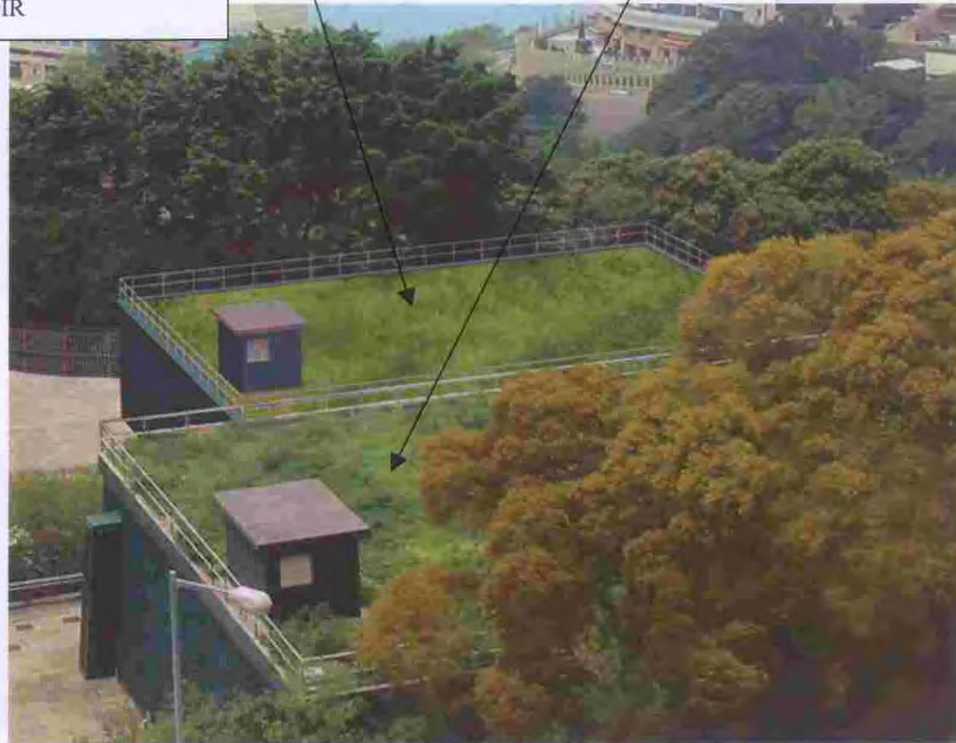
擬建華富海水配水庫 PROPOSED WAH FU SALT WATER SERVICE RESERVOIR
