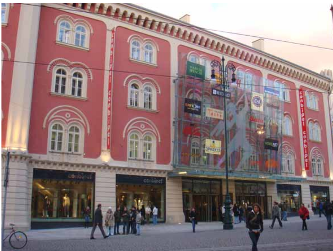
The Palladium in Namesti Republiky where a 19th century barrack has been refurbished into a multi-purpose commercial development
