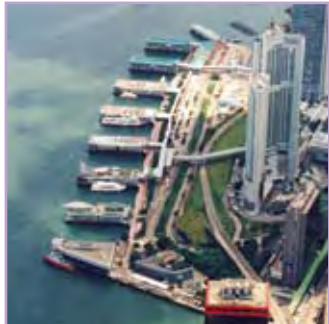
Site 1 near Central Piers No. 4 - 6
