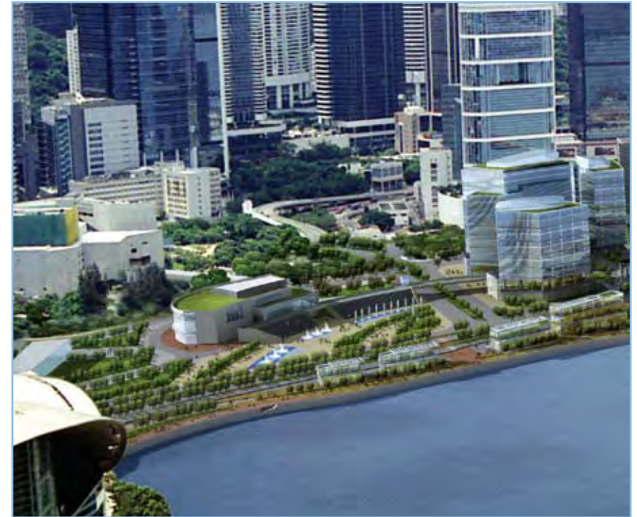
Aerial View of Sites 5 and 6
