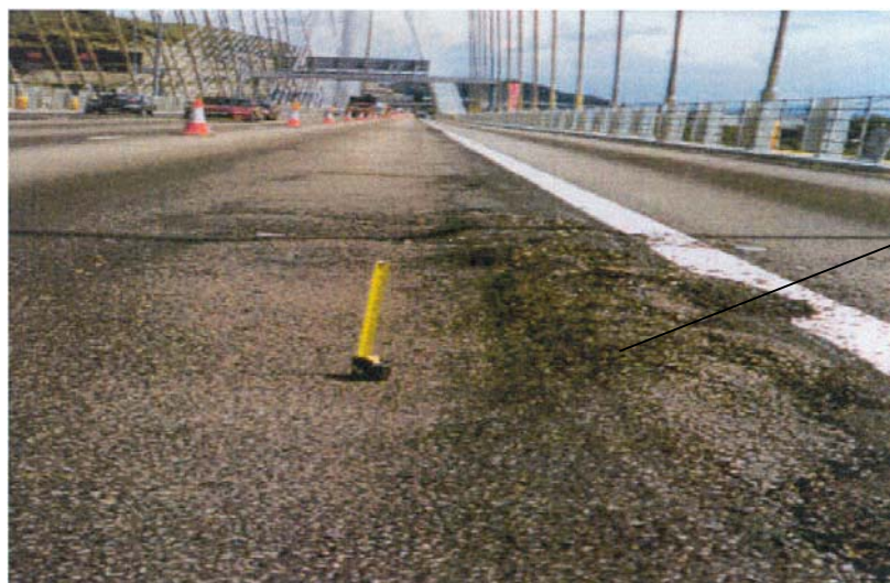
Figure 2 – Premature deformation of asphalt surfacing at Ting Kau Bridge
