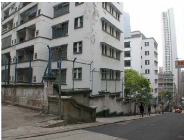
Boundary wall along Aberdeen Street
