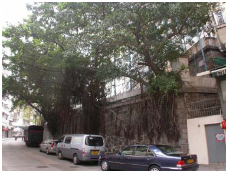
Retaining wall along Hollywood Road
