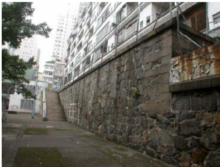
Retaining wall and flight of steps on the lower platform
