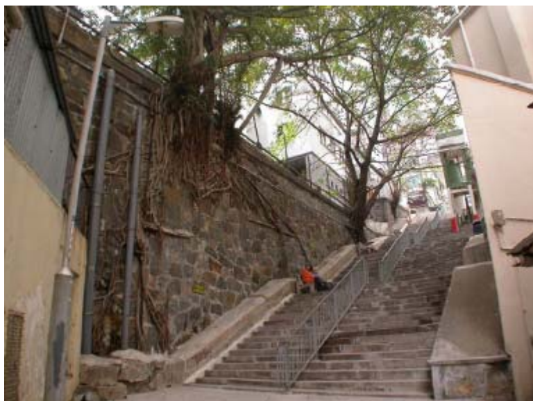
Retaining wall along Shing Wong Street
