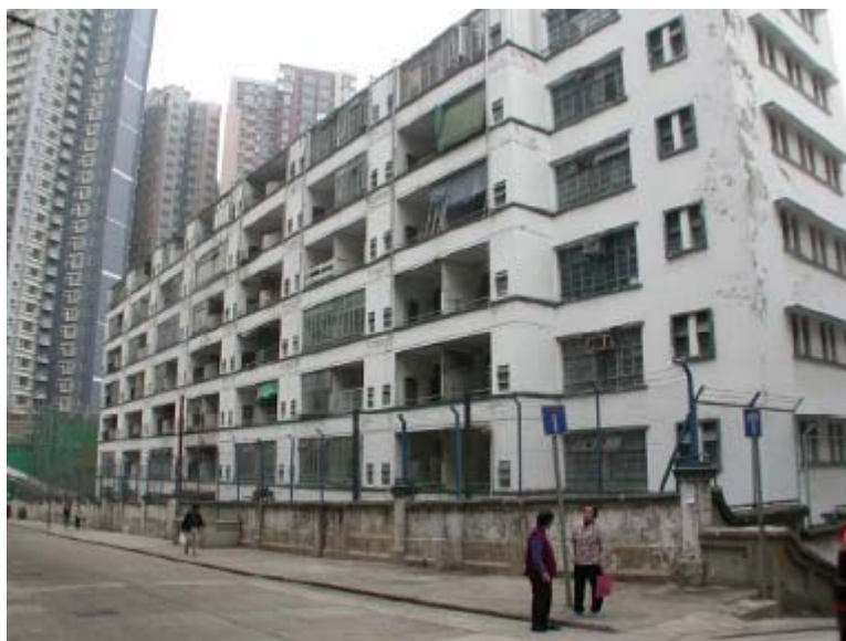
Boundary wall along Staunton Street
