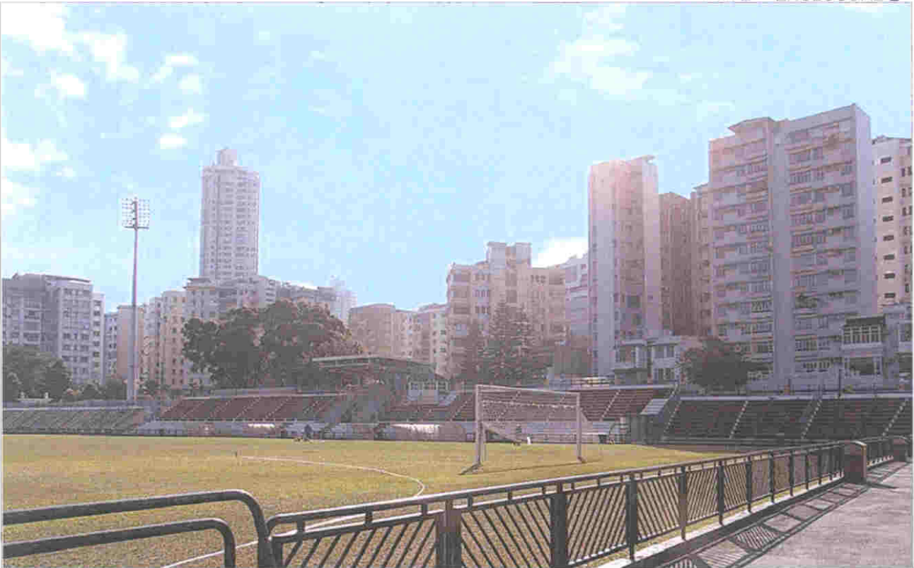
旺角大球場改善工程 - 望向球場南面看台 (工程前) Improvement Works for Mong Kok Stadium - View of Stadium South Stand (Before)
