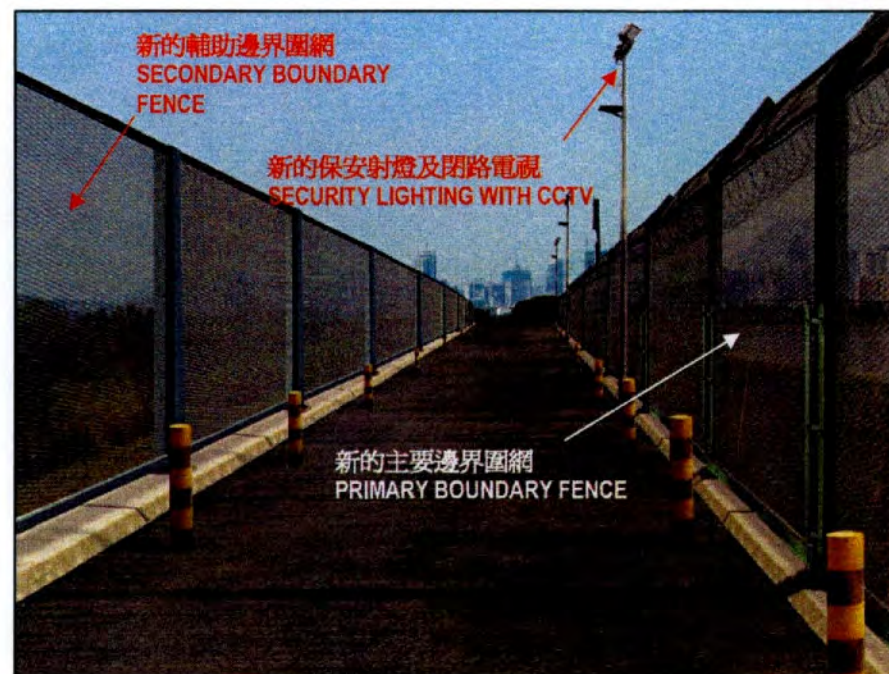
新的邊界巡邏通路和主要及輔助邊界圍網 NEW SECTION OF BOUNDARY PATROL ROAD WITH PRIMARY AND SECONDARY BOUNDARY FENCES
