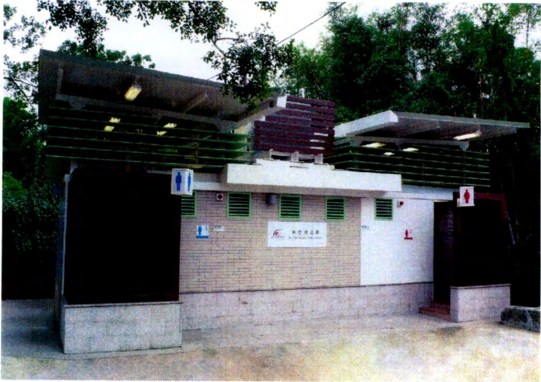
廁所改善後之外貌 EXTERIOR VIEW OF TOILET AFTER IMPROVEMENT
