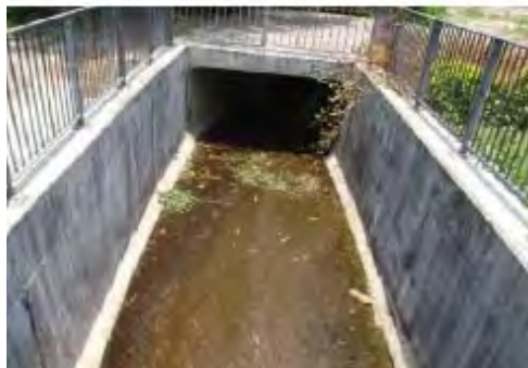
排水渠 Drainage Channel
