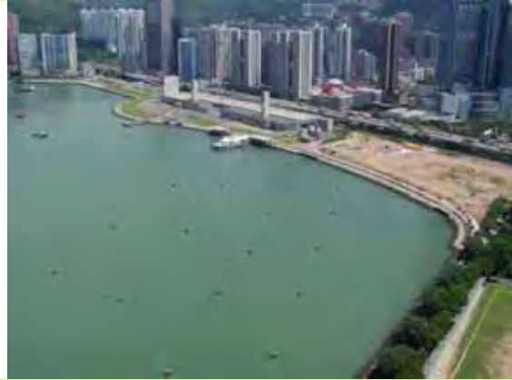
After rectification in July 2006
