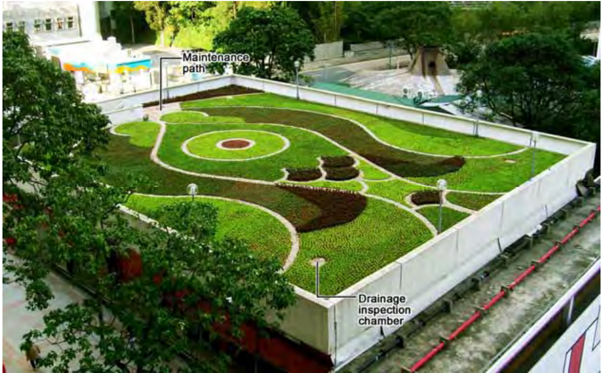
Completed green roof – side view
