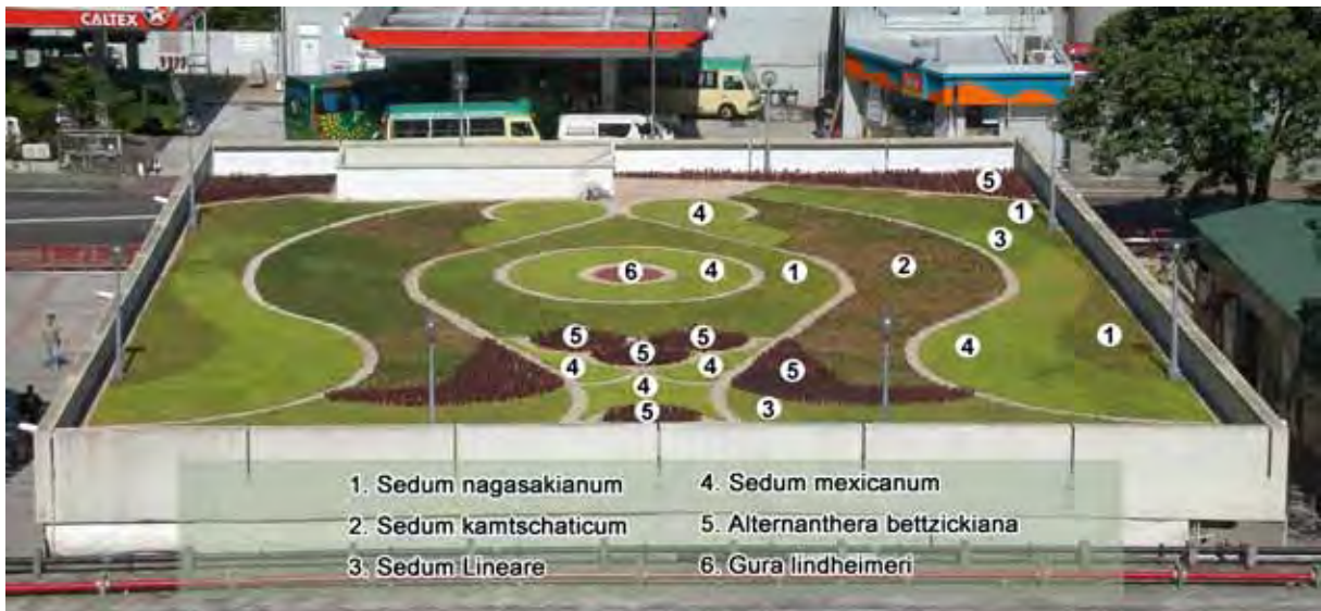
Completed green roof – front view and planting layout
