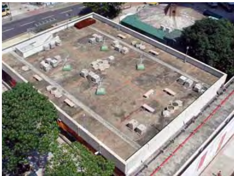
Rooftop of market before greening
