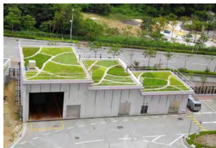
Fanling Area 36 Phase 1 & 2
