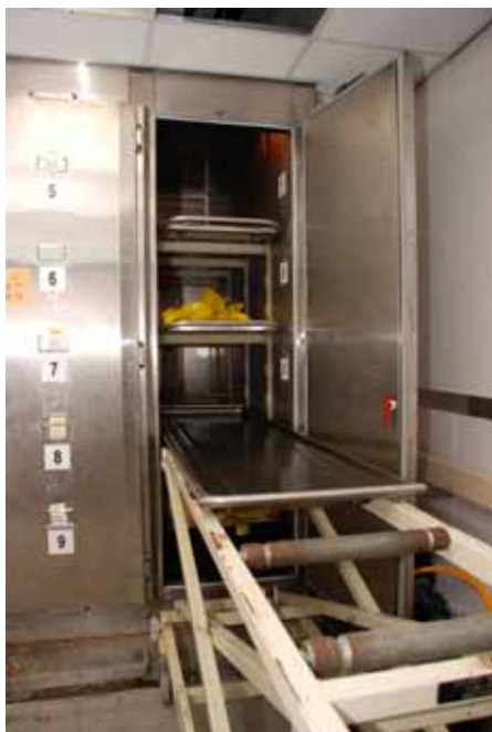
Photo 3 and 4 : Special compartments designed for deceased babies and large sized adult bodies
