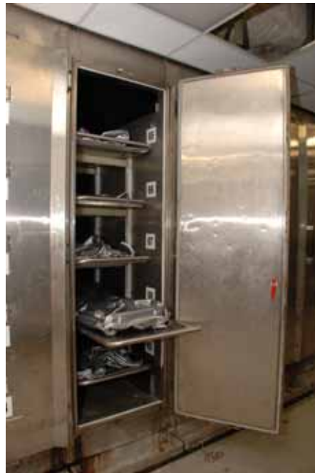
Photo 2: Typical mortuary compartments
