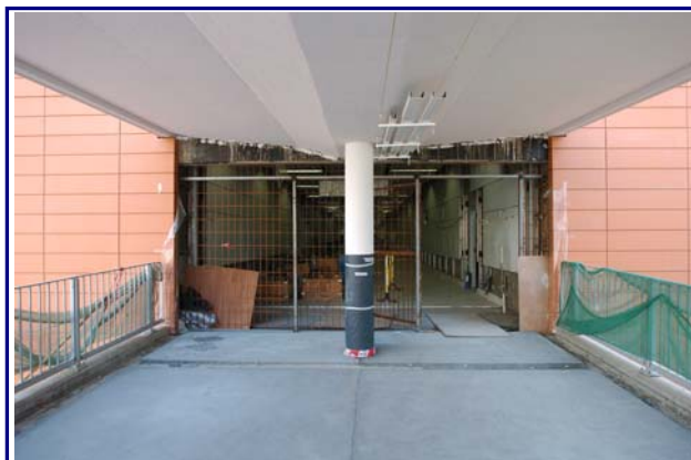
The northern end of Austin Station is connected to Jordan Road Footbridge
