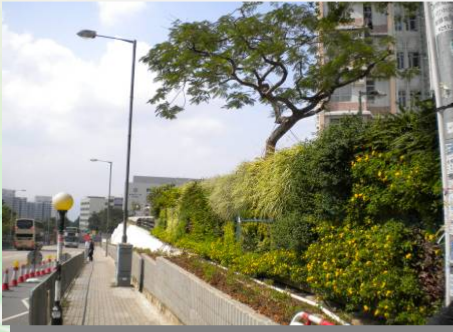
秀茂坪南邨 大面積固定綠化板作 隔音屏障 Sau Mau Ping South Estate Vertical Green Panels as Noise Barrier
