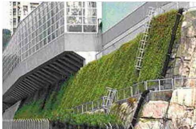
油麗邨一期的人造斜坡試用綠化噴播方法 Mulching Method at Yau Lai Estate Phase 1
