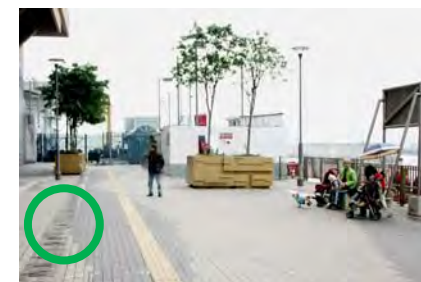
Raised and loosely scattered planters cannot perform shading and greening functions (Grand Promenade, Sai Wan Ho)
