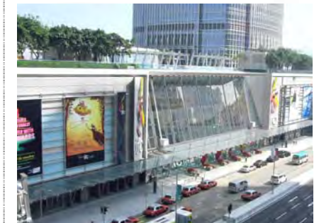
No visual connection with the ground (Hong Kong Station Development, Central)
