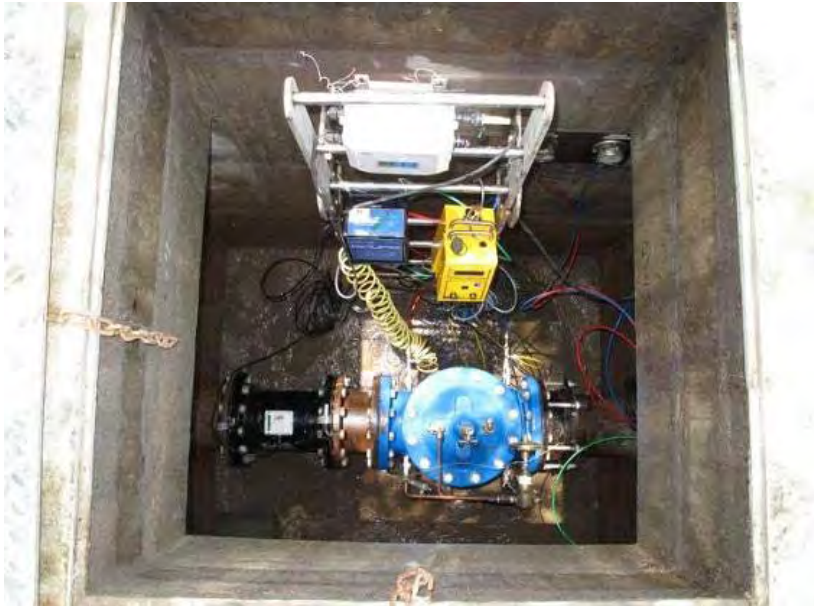
Pressure Reducing Valve and Flowmeter
