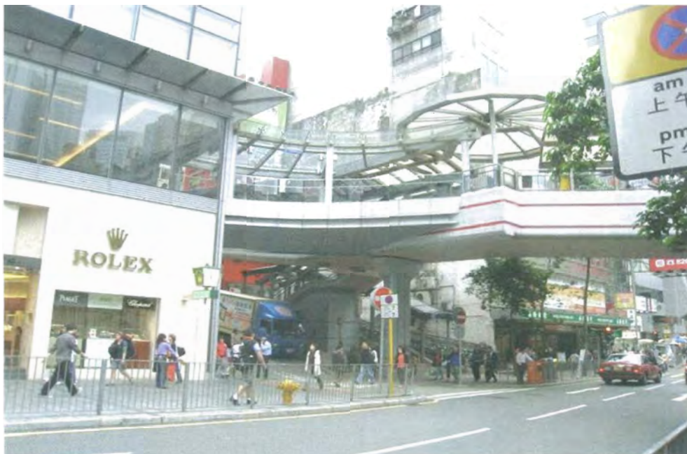
Photo 9.4: By reprovisioning the escalator within the building, a much more spacious pedestrian environment is created at ground level.
