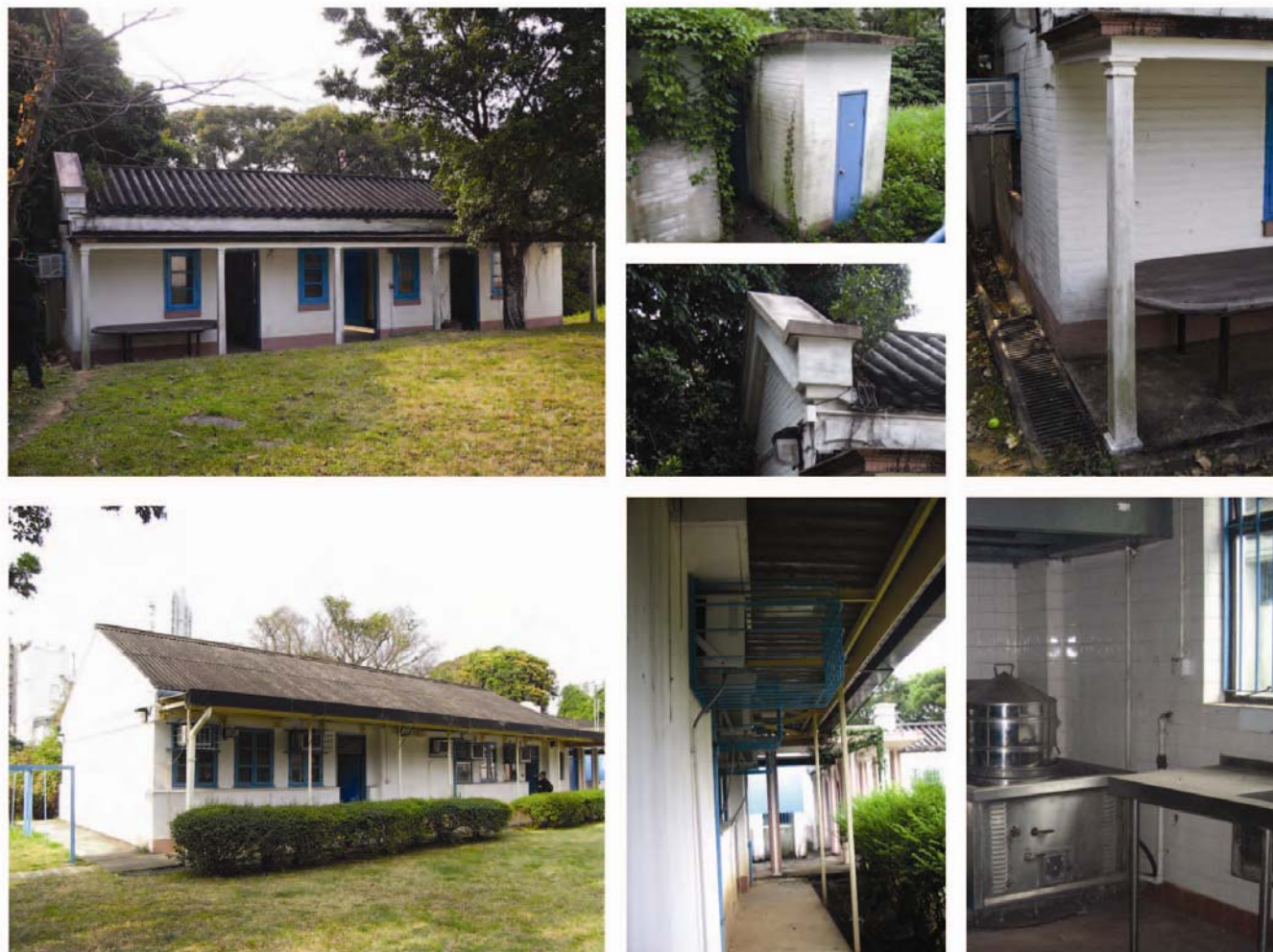
Existing Buildings 樓宇現貌
