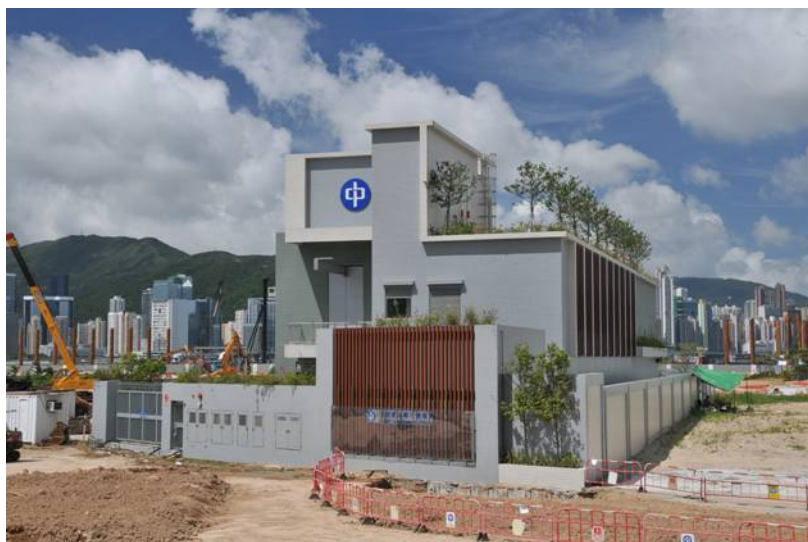
啓德郵輪碼頭變電站 Kai Tak Cruise Terminal Substation
