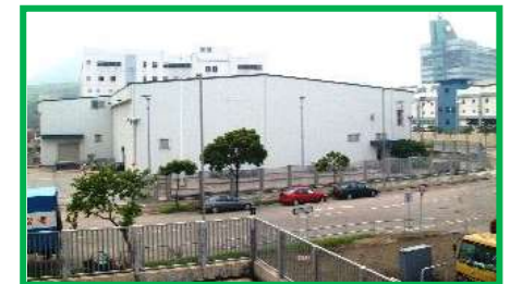
Submarine cable landing
