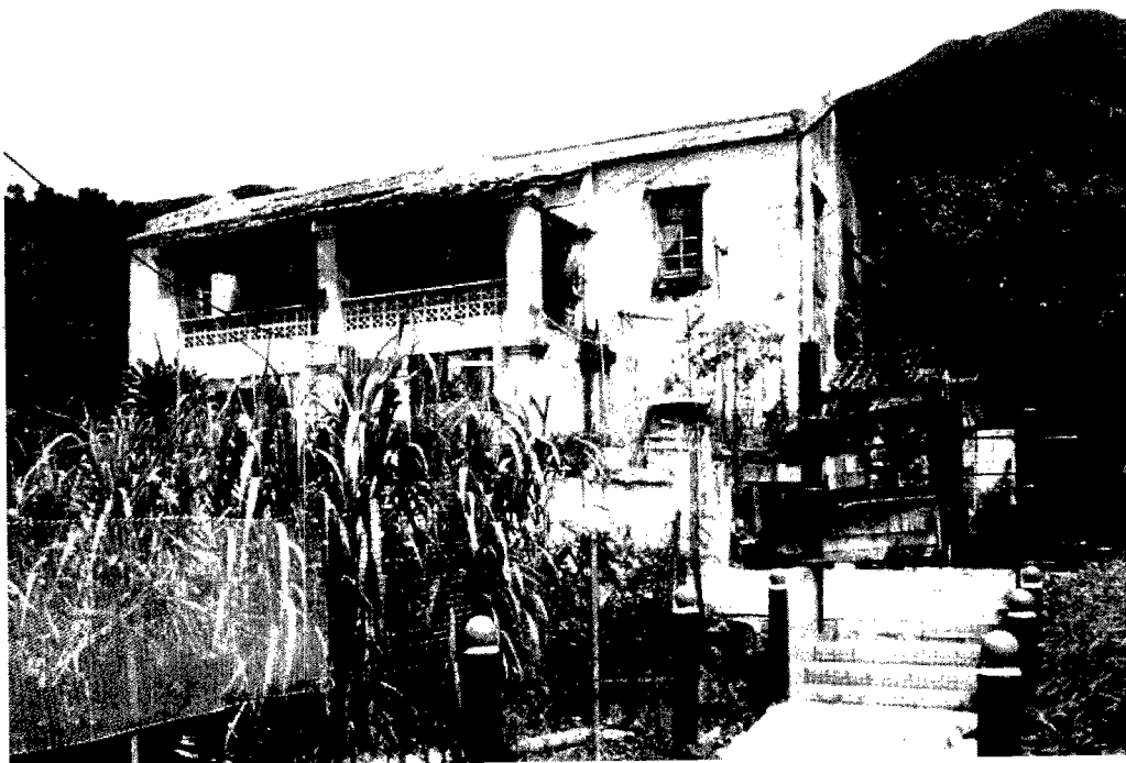
Existing Condition of Hung Lau
