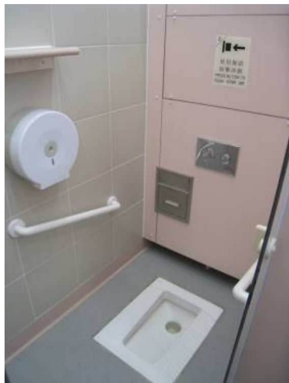
After conversion 改建後
