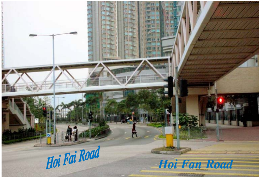
Footbridge at the junction of Hoi Fan Road and Hoi Fai Road in Tai Kok Tsui
