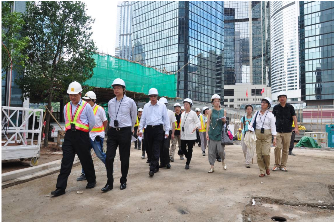
Members visit the site of the new LegCo Complex to gain a better understanding of the traffic and transport arrangements for access to the Complex.
