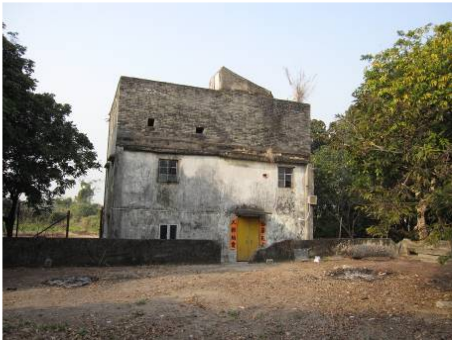
Front elevation of the Building
