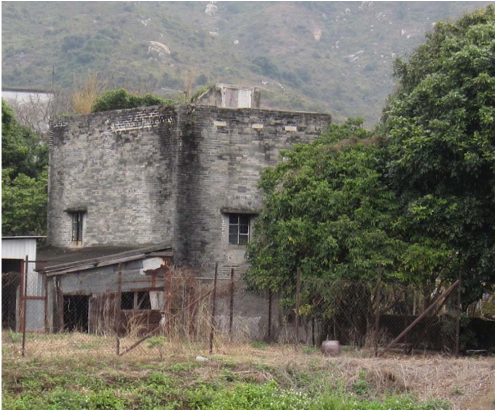
North elevation of the Building
