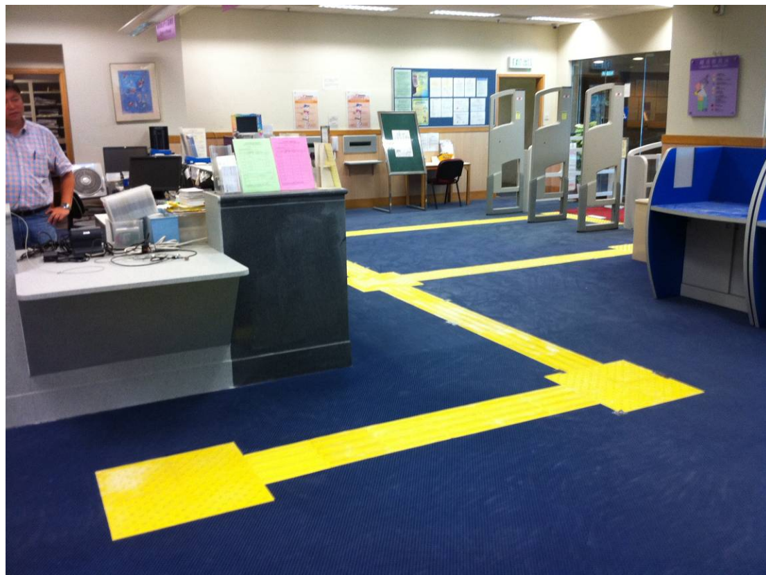
改善觸覺引路帶(Improve tactile sign/guide path)
