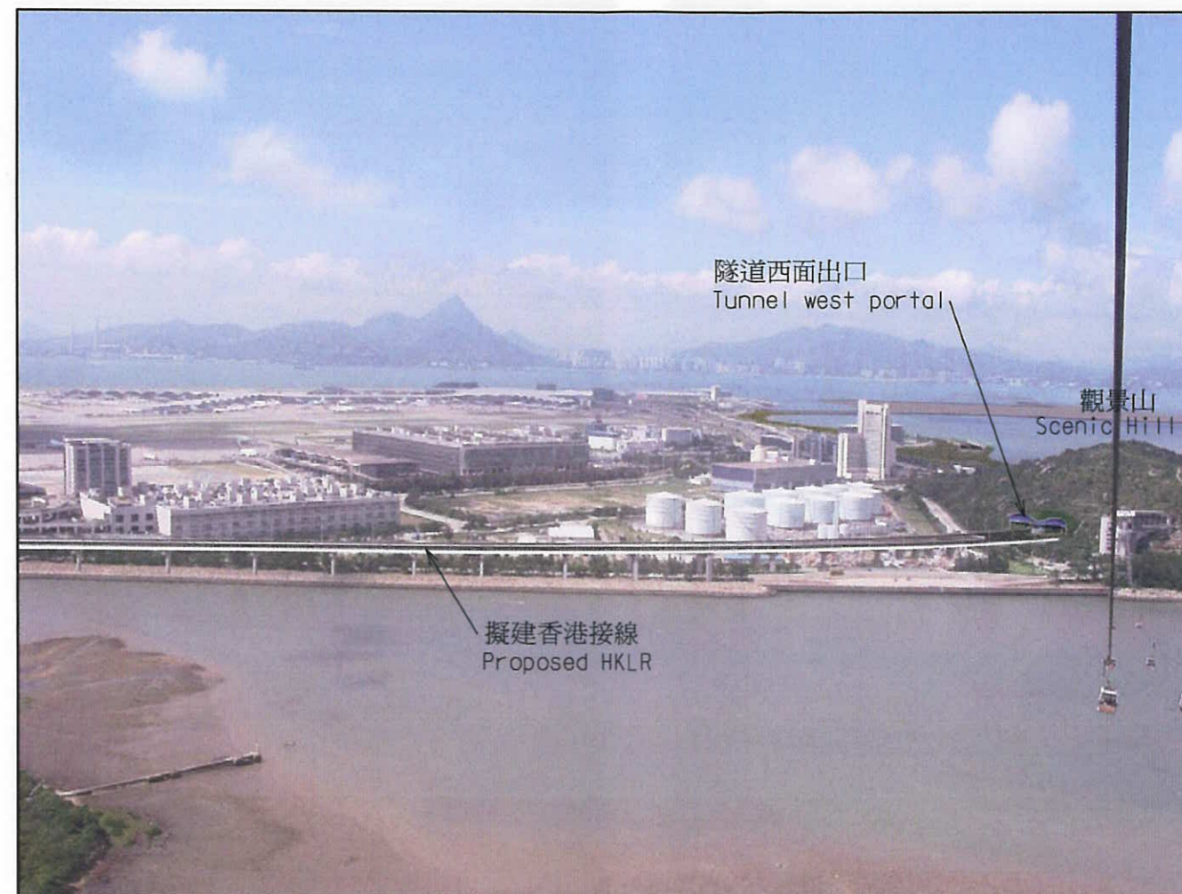
視圖2 - 香港接線沿機場島海堤至位於觀景山之隧道西面出口 View 2 - HKLR along seawall of Airport Island to tunnel west portal at Scenic Hill
