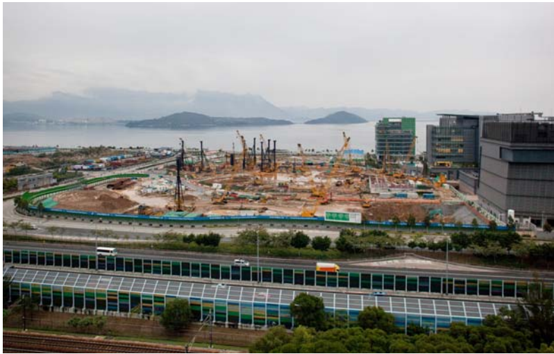
Piling work started in Hong Kong Science Park Phase 3
