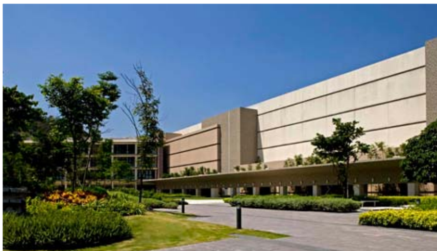
High-end data centre operating in Tseung Kwan O IE
