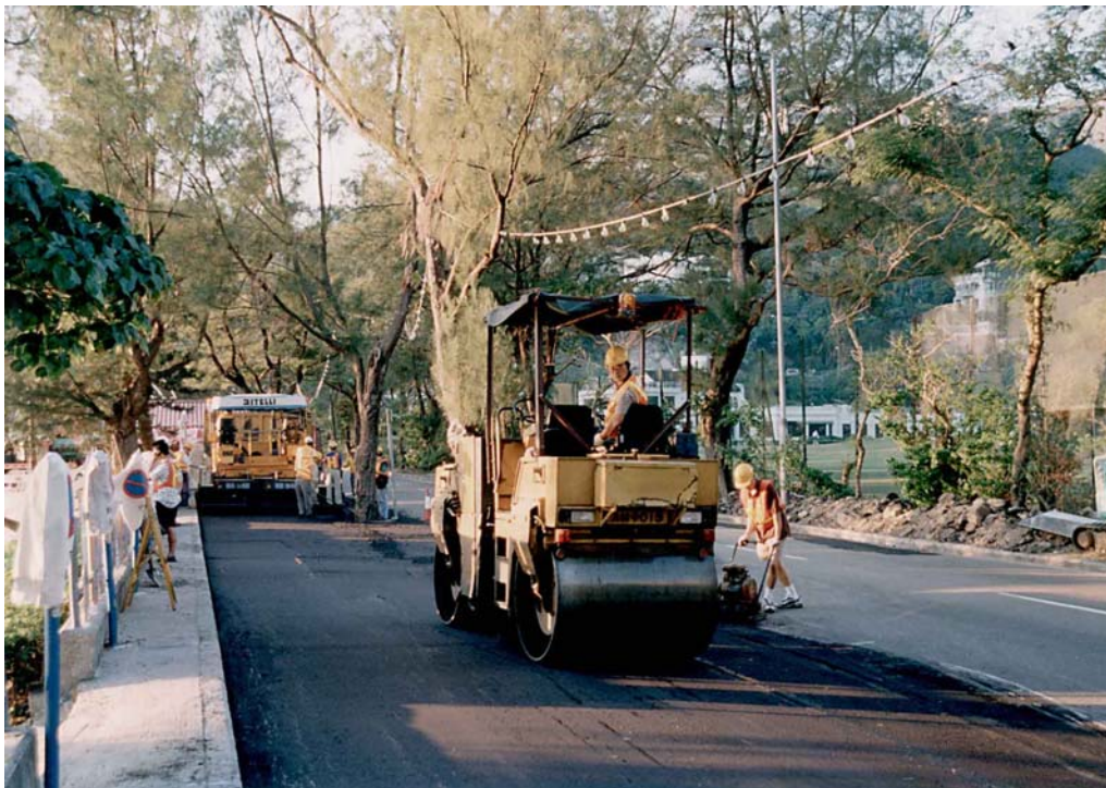
[Figure 2] Traditional repair method for bituminous pavements – Laying and compacting new bituminous materials
