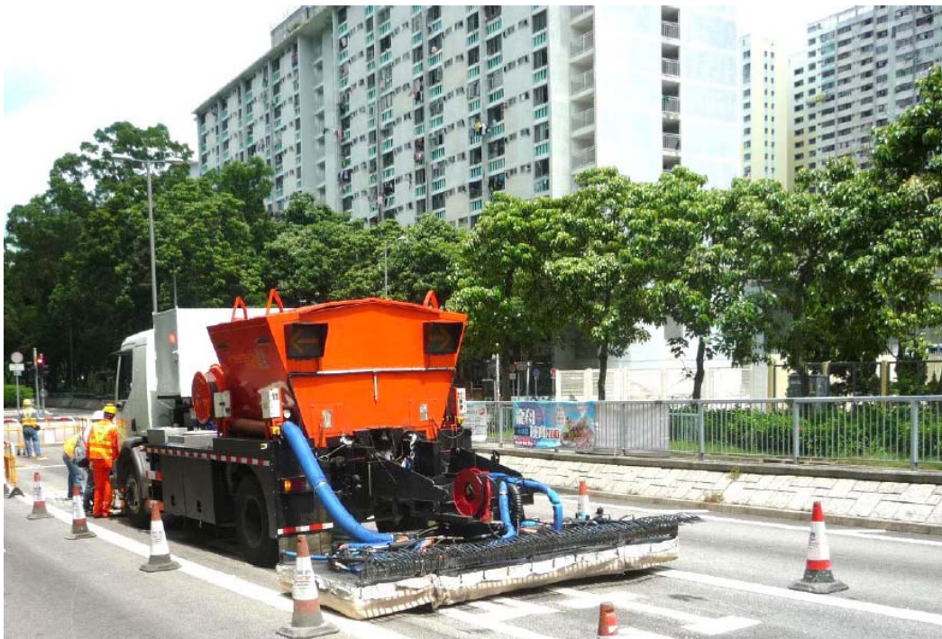
[Figure 4] Pavement resurfacing by large-size thermal patcher
