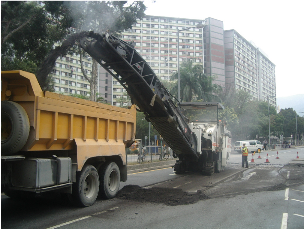
[Figure 1] Traditional repair method for bituminous pavements – Cold milling of defective materials
