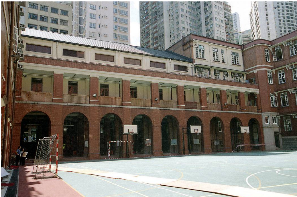
View of east wing of the school building from the school playground
