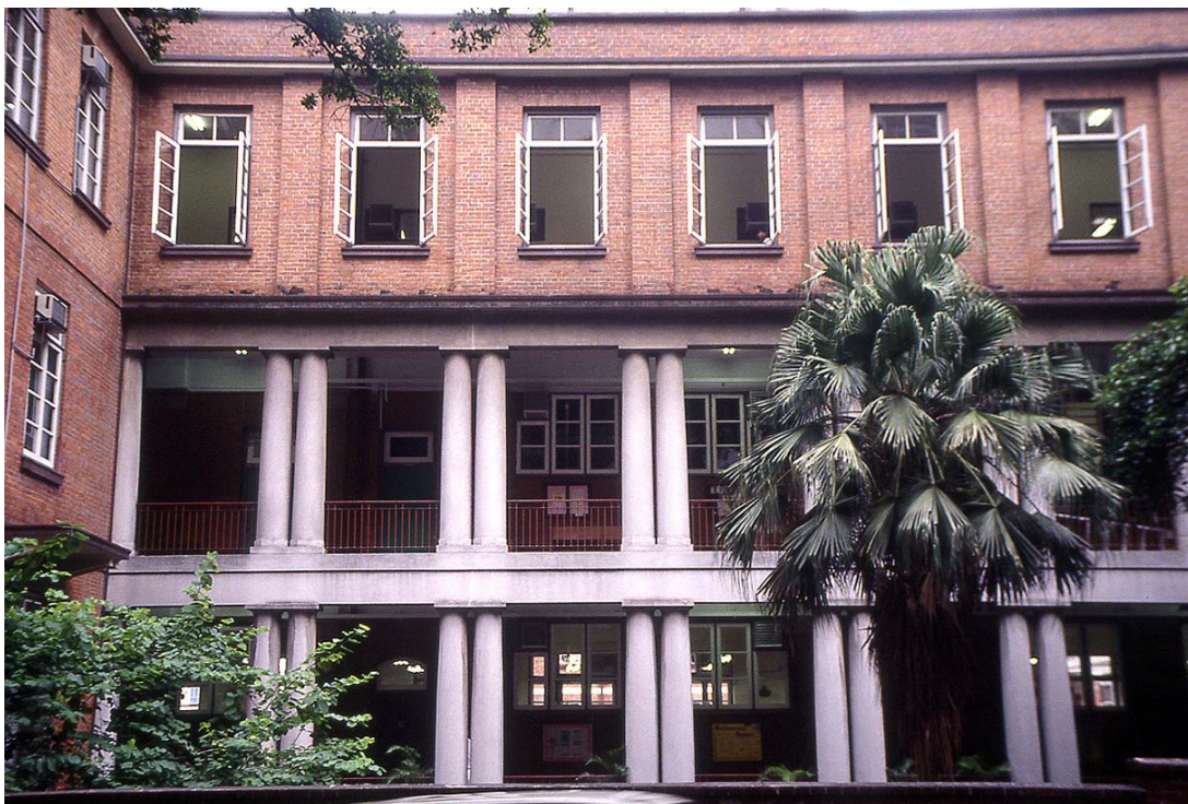
View of south wing from Bonham Road
